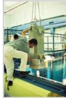
Fig. 3: Transfer system for TN-MTR dry loading at RR site
